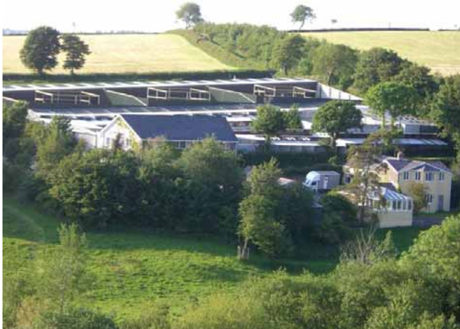
Part of the IWC facility in Wales.
